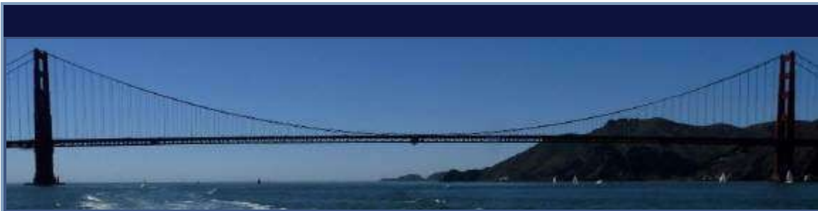
Golden Gate Bridge
